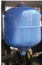
5 gallon oil make up system
