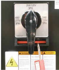
Multi-Voltage selector switch with lockout
